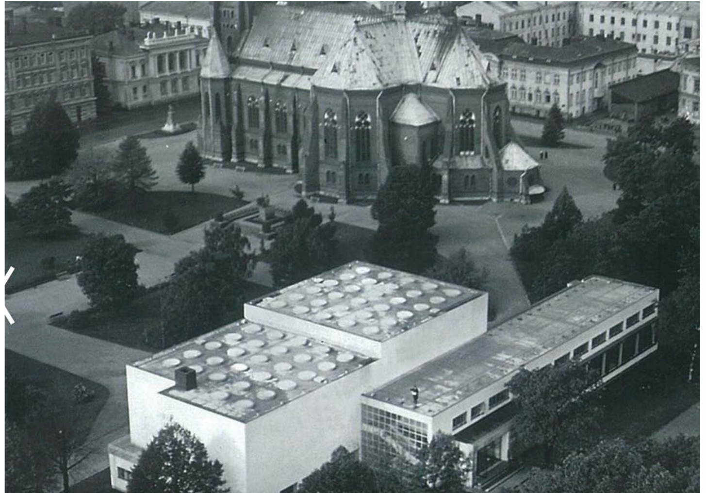
Pre-1940 photograph of the library adjacent to the Viipuri Cathedral
